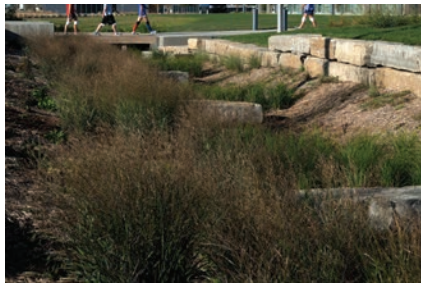
A series of bioswales, constructed wetlands, restored prairie and walking trails recreate natural environment areas that also process storm water.
