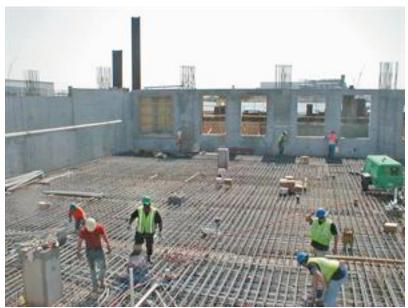
Here note the lack of special rebar placement, joint doweling, or joint detail construction. Savings on these special construction items, along with the time savings of a monolithic placement, helped to bring this stage of the project in on time and below budget.
