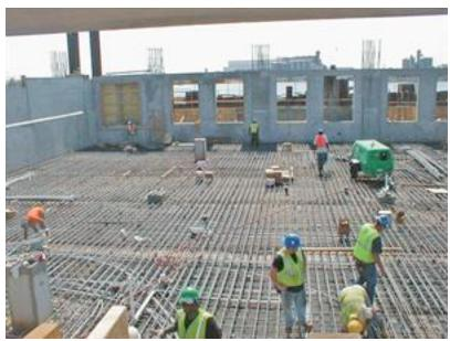
Continuous rebar in this 110x200-ft. 7- to 11-in. slab on grade will provide restraint against concrete expansion allowing the contractor to place a monolithic slab without any contraction joints, seams, or shrinkage cracks. The resulting slab will have greater durability and save the owner slab and joint maintenance cost.
