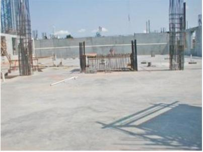
The finished slab provides a uniform surface without any shrinkage cracks or contraction joints. The slab was constructed by adding, a shrinkage-compensating component, to a standard concrete mix to create shrinkage-compensating concrete in accordance with ACI 223R10, "Guide for the Use of Shrinkage-Compensating Concrete."
