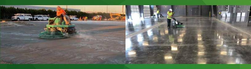
IceStart™ is a Surface Applied SCM (Supplementary Cementitious Material) Admixture that is the first treatment of a Two-part Surface Applied Admixture Cure and Densification System, called GreenIce Cure System™ with GUnanoInside technology— that is designed for Interior or Exterior concrete. Used only @EarlyAge concrete staging, it is a chemical and mechanical process applied at time of concrete placement and power troweling.
