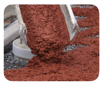
**Materials:** Green Umbrella Integral ColorPac colors do not contain fillers or extenders. All pigments are permanent, light-fast, inert and stable to atmospheric conditions. GU Integral ColorPac colors comply with ASTM C979, Pigments for Integrally Colored Concrete. Integral colors are *not* designed for dust-on application.
