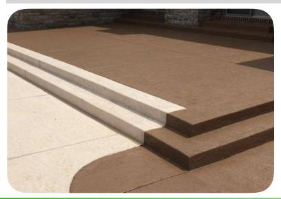
**Job Site** - GU Integral ColorPac Integral Color can also be added at the job site. Add bags to drum and mix for 12-15 minutes (120-150 revolutions). Order concrete at a workable slump (3-5") and always keep water addition to a minimum. Make every effort to maintain consistency with multiple loads. Water addition can lead to inconsistent color.
