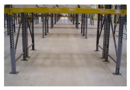
Fig. 4. Workplace safety: white concrete floors work well in industrial settings, too. The light color reduces shadows and improves lighting efficiency in large buildings, such as warehouses.
