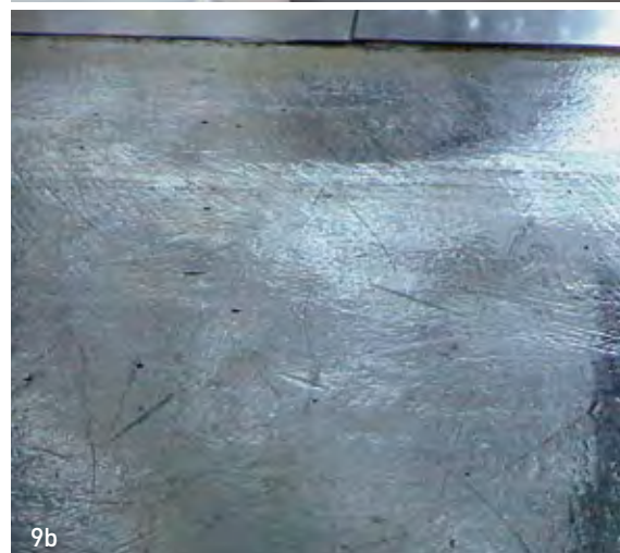
Figure 9 Cafe with burnished concrete floor (plus sealer) 9a → Steel trowelled burnished finish over majority of floor 9b → With some areas displaying trowelling marks
