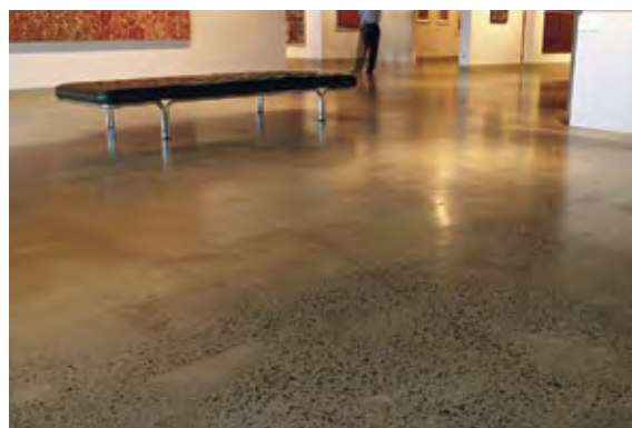
Figure 51 Existing floor ground to remove previous finish and expose the aggregates. Cracks, uneven aggregate exposure, repairs and different concrete colours rather than detracting, may add to the attractiveness of the finish. Art Gallery of New South Wales
