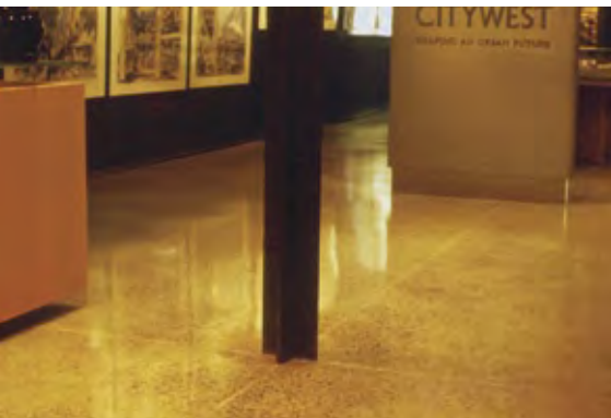
Figure 46 Saw cut joints in line with columns
