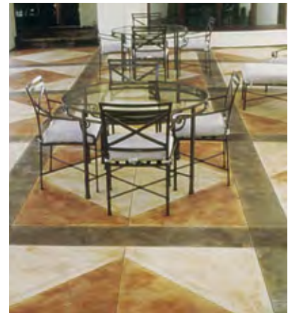
Figure 21 8 Patterns can be formed with shallow saw cuts and colours. Saw cuts are also used to create boundaries for application of chemical stains
