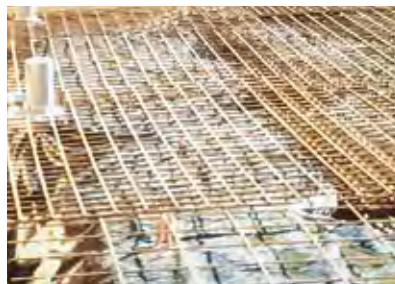
Figure 44 SL81 mesh used to control shrinkage cracking in polished section of residential floor slab.
