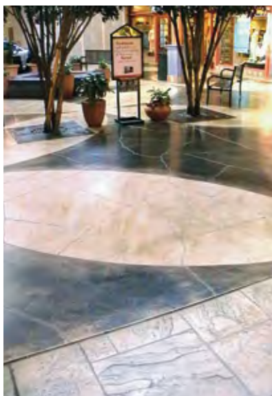
Figure 50 Random stone patterns have been formed by cutting joints in the thin 10-mm-thick topping to existing slab. Pattern can be used to conceal any random cracking in the existing slab
