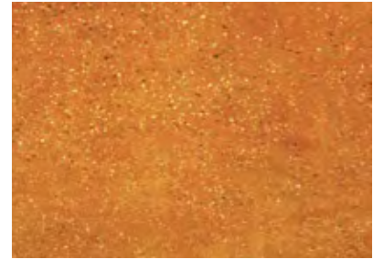
Figure 40 Uneven aggregate distribution caused by use of immersion vibrator
