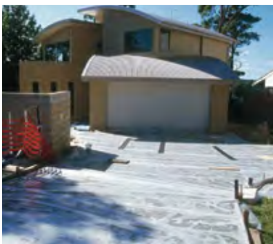
Figure 43 Clear plastic sheeting used for external applications
