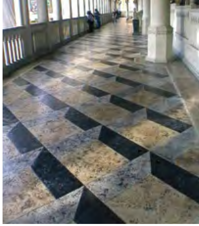
Figure 14 Chemically stained concrete floor providing three-dimensional appearance
