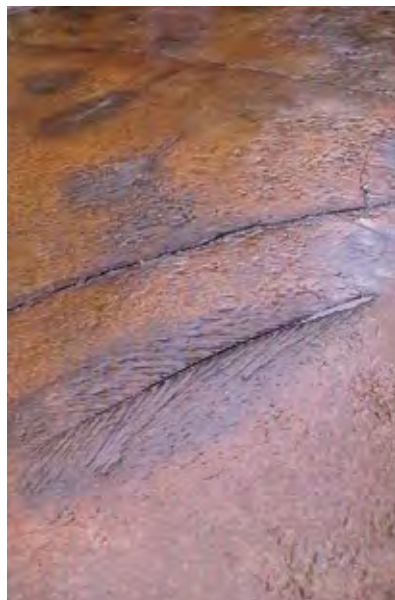
Figure 25 Shallow texture with palm frond pattern imprinted into the surface. Coloured using chemical stains
