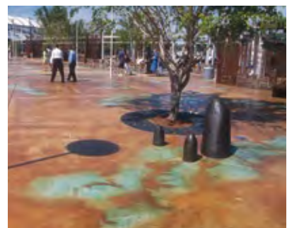
Figure 36 External polished pavements can have adequate slip resistance. Sydney International Airport
