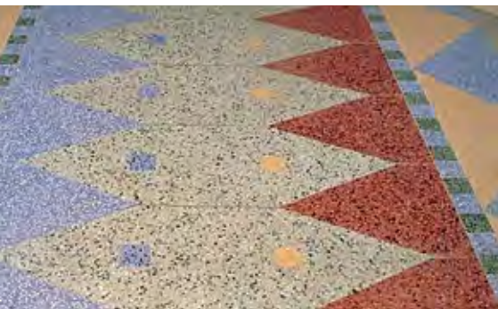
Figure 6 Coloured terrazzo finish incorporating coloured marble chips as aggregate and inorganic mineral (metal) oxide pigments. The lighter coloured areas are unpigmented. Epping Plaza Shopping Centre, Victoria (reproduced with permission from Ability Chemicals)
