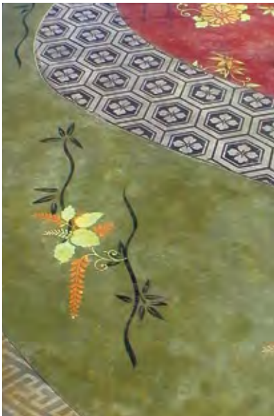
Figure 18 Dyes/tints used where strong vibrant colours were required to highlight details. Chemical stain used for the mottled green background.
