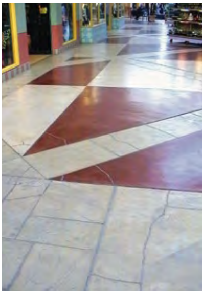
Figure 34 10-mm-thick topping with textured/patterned surface in shopping centre
