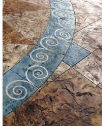
Figure 26 8 Patterns produced by colouring the concrete then abrasive blasting selected areas through stencils to remove some/all of the coloured surface material. This changes the texture and creates surface features.
