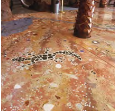
Figure 29 Artistic terrazzo incorporating various materials and features. Materials include coloured glass, PVC pipe sections and pieces of coloured marble. Artist: David Humphries of Public Art Squad
