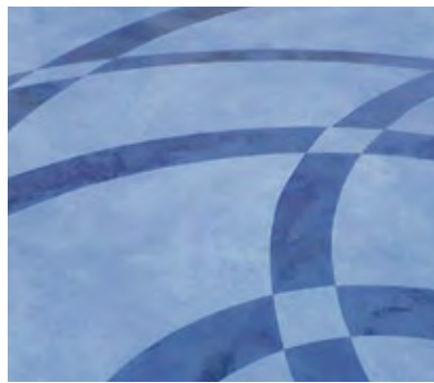
Figure 35 Thin cementitious polymer topping about 10-mm-thick with darker areas consisting of a blue-coloured cement-based micro-topping about 1 mm in thickness. Surface was finished using a solvent-based blue dye. Pattern formed using self-adhesive stencils.
