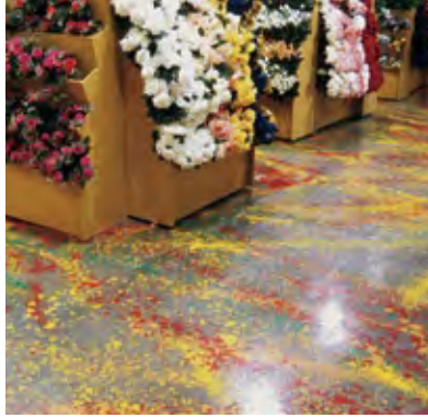
Figure 19 Paint system used to provide decorative finish to existing floor
