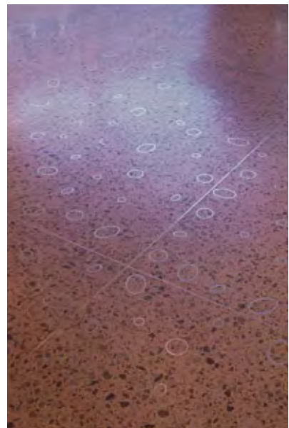
Figure 28 Cast-in stainless steel inserts used to add interest. Shapes formed by cutting pipe at various angles
