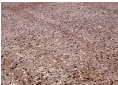
Figure 10 Hard aggregates can provide a decorative finish having a durable and wear-resistant surface.
