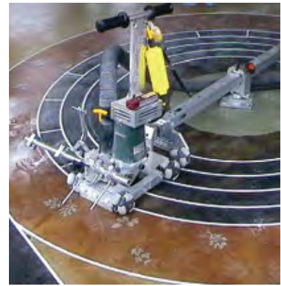
Figure 15 Pattern lines should be cut using guides to ensure accuracy
