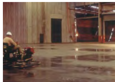
Figure 8 Burnishing the concrete by extended trowelling (areas with gloss appearance completed)
