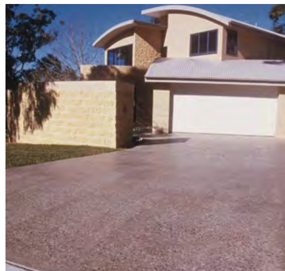
Figure 5 Driveway with ground finish incorporating decorative white quartz aggregate and 1% green pigment
