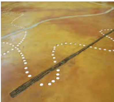
Figure 30 Bronze artwork and ceramic tiles embedded into existing floor with colour added to surface. Tiles placed in shallow cored holes and surface coloured by applying slurry of pigment to existing slab.
